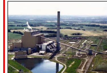
Transalta Canada - >200 MWe Chilled Ammonia - Coal
