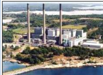
EoN Karlshamn Sweden - 5 MWth Chilled Ammonia - Fuel/Gas
