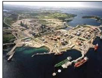
Statoil Mongstad Norway - 40 MWth Chilled Ammonia - Gas
